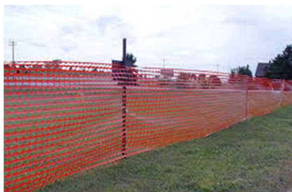
Example 2: Installed hazard fence
